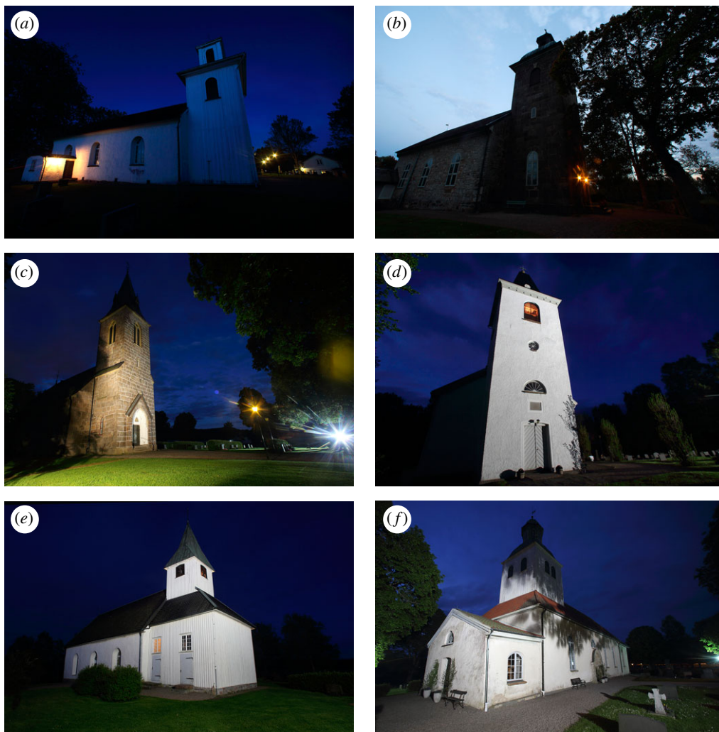
Figure 1. Examples of the three categories of flood-lighting used on the churches examined during this survey; (a,b) not lit, (c,d) partly lit, (e,f) fully lit. All churches shown harboured colonies of long-eared bats in the 1980s. In 2016 the colonies were gone from (d) and (e) but remained in (a–c) and (f).
