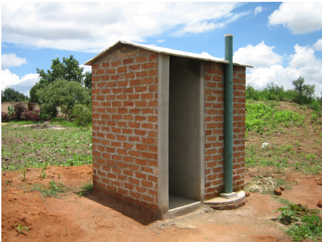
Fig 1. The Blair VIP latrine. Simple construction of ideal family latrine used extensively in Zimbabwe. Often used also as an ablution facility as well as a latrine; this is adapted for individual family use. The flue (vent) exhausts the odour and also diverts flies. The pit is approximately 5 m deep. Photograph: Dr. Peter Morgan.
