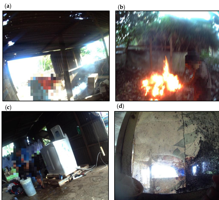
Figure 2. Risk factors and behaviours observed in the home environment that increase the risk of injury or harm to children: (a) Cooking on an open fire in a cooking shed filled with smoke. Low-quality building materials used in structure; (b) Child burning rubbish and standing near flame; (c) Electrical extension blocks and power cables next to a washing machine and in the vicinity of a water spill; (d) Fabric covered in mould next to a food preparation surface.
