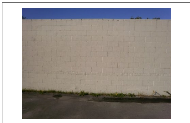
Figure 3. Impenetrable Brick Wall.
