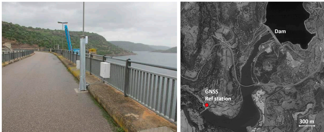
Figure 3. One of the GNSS antenna monitoring the dam and the position of the reference station.
