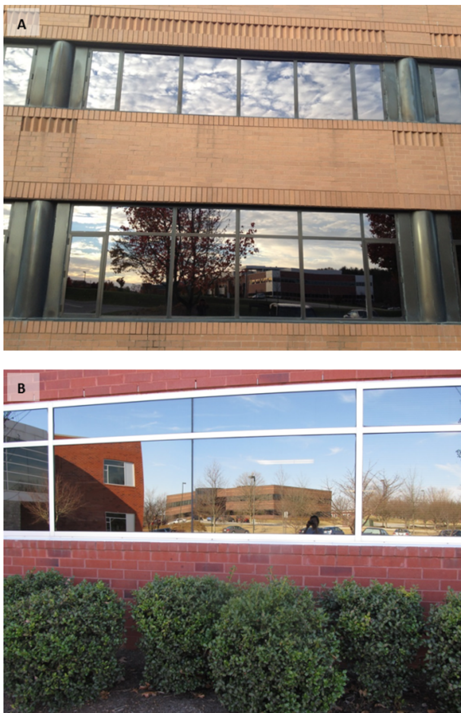
Figure 2 VTCRC windows. Typical highly reflective windows at the VTCRC, Blacksburg, VA (A) Building 2 (B) Building 15.
