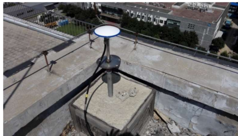
Figure 5. Surrounding environment of the antenna installed on the roof of the Academy of Opto-Electronics for the zero-baseline experiment.
