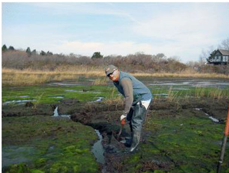
Fig. 5. Example of a hand dug runnel (0.15–0.2 m wide by 0.2 m deep) to drain the high marsh. Photo taken by W. Ferguson
