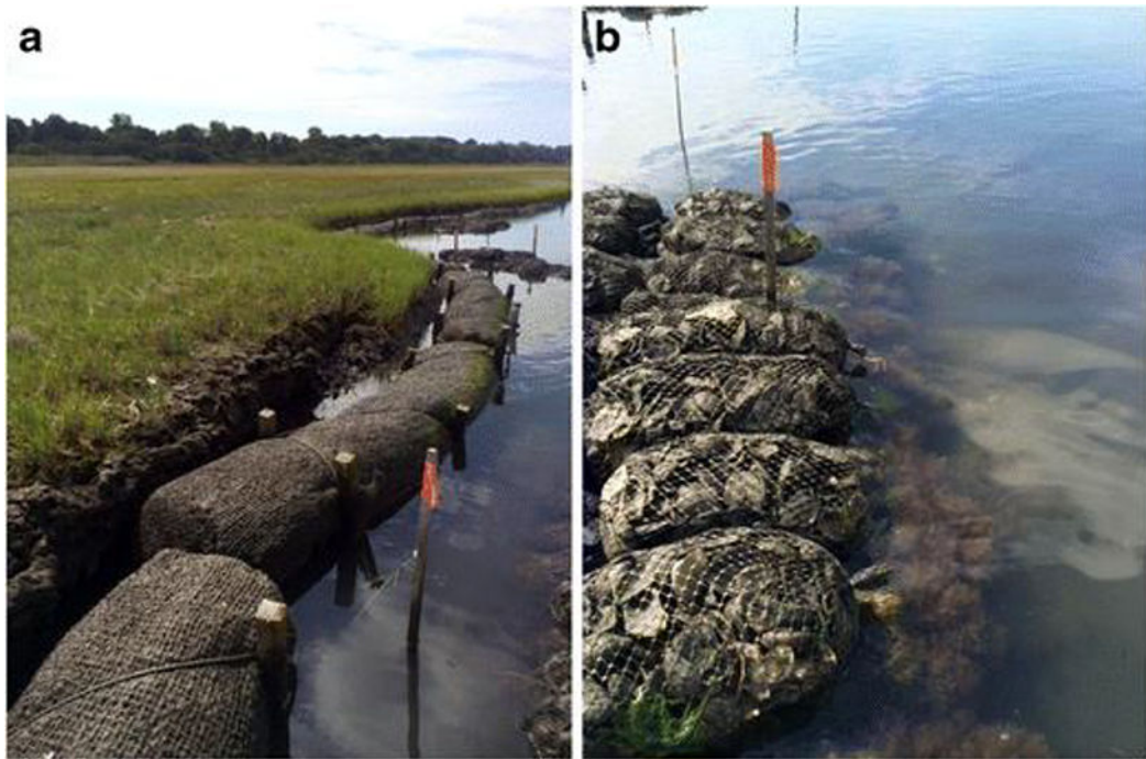
Fig. 4. a Coir logs set along the Narrow River shoreline b Bags of oyster shell set along the NRE shoreline Photos taken by C. Vandemoer
