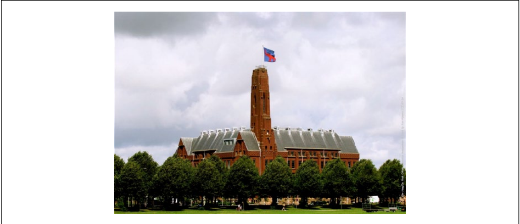
Figure 31. The former Exxon headquarter in The Hague nicknamed “The Red Elephant.” Source: Roel Wijnants.
