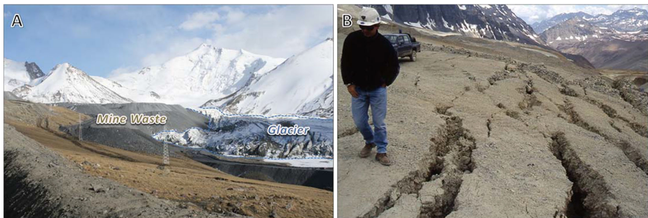
Fig. 3 a Mine waste dumped on the margin of the Davidoff Glacier at Kumtor Mine, Kyrgyzstan, causing deflected and accelerated flow of the glacier in response to the additional loading from the mine waste. b Example of cracking caused by ice creep affecting a haul road constructed over a mine-waste-/debris-covered glacier at a copper mine in the Central Andes, Chile
