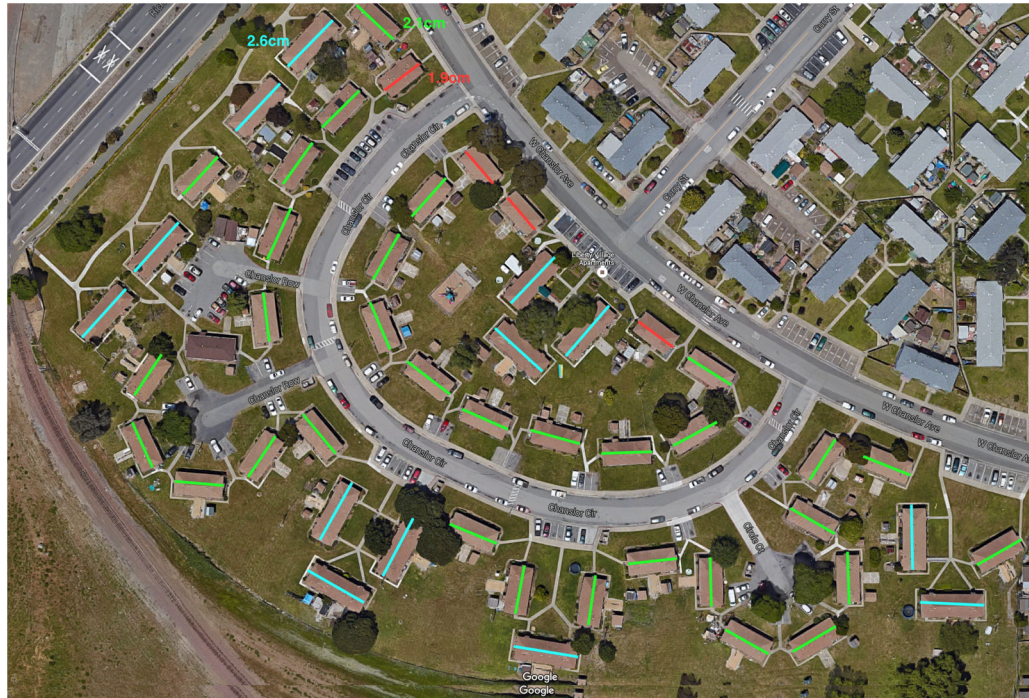
Figure 5. Measurements of the rooflines of the buildings in Liberty Village. Three measurements found: red was 1.9 cm, green was 2.1 cm, and blue was 2.6 cm. Red lines show duplexes with 2 one-bedroom units. Green lines show duplexes with 2 two-bedroom units. Blue lines show duplexes with 2 three-bedroom units. In total, there are 100 units.
