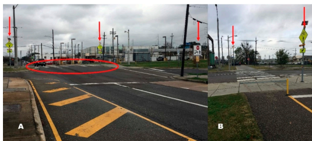
Figure 2. Crossing equipped with rectangular rapid flash beacon as seen from the perspective of (A) motor vehicle user and (B) greenway user.
