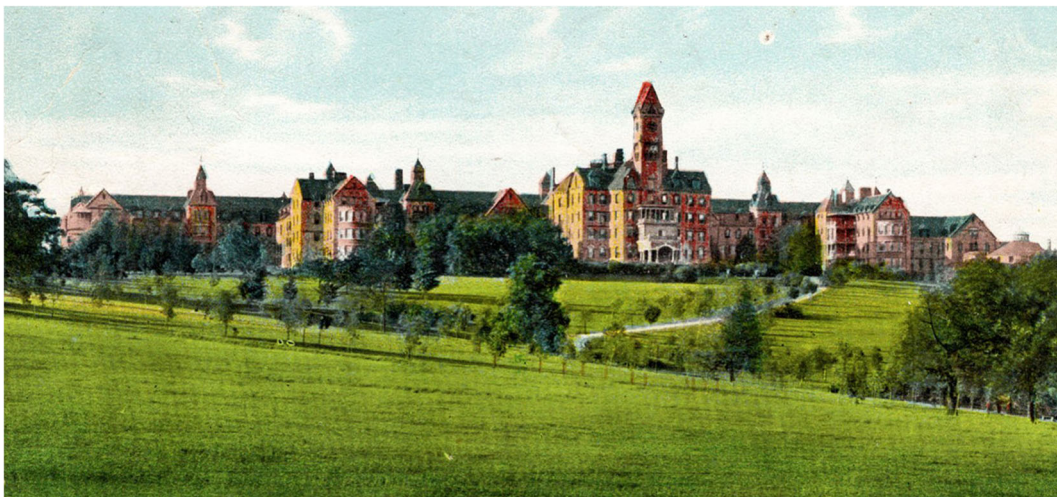
Figure 1 Kirkbride Hospitals were built at many locations in the Midwest and Eastern USA, emphasizing the positive effects of natural sunlight and air available in a country setting. A number of these facilities have been demolished including the one illustrated here: The Bloomingdale Asylum in Massachusetts (Image Credit: John Michael Currie, FAIA, FRSPH).
