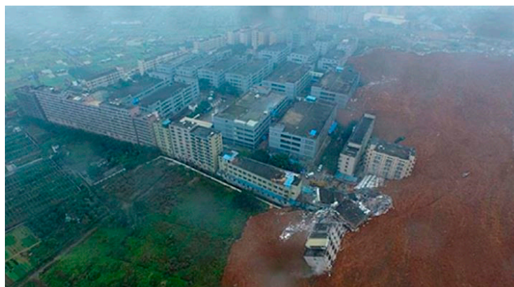
Figure 5. C&D waste landfill landslide in Shenzhen, China [105].
