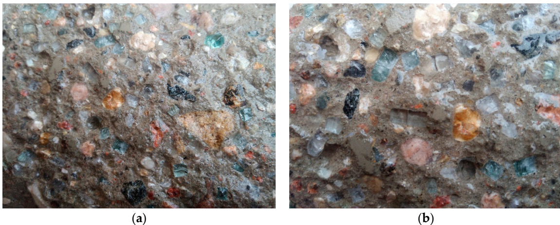
Figure 10. The fracture surface of the RGA concrete: (a,b) various fragments of the surface.
