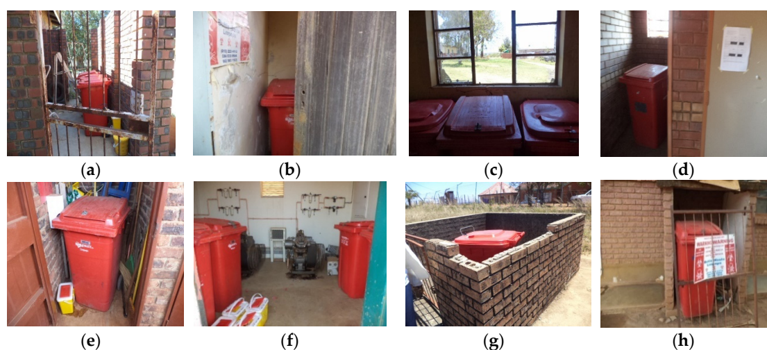
Figure 6. Photos taken by researcher during field work showing central storage areas for HCRW in Vhembe District Healthcare Facilities: HCRW storage rooms with doors, but, without locks (a,b); HCRW storage room without a door (c); HCRW stored in the same room with cleaning and gardening equipment (d); HCRW storage room with a broken window (e); an old incinerator room converted to storage area (f); HCRW storage area with a gate, a low fence but, without a roof (g); HCRW being stored by the corner of a wall, not in a secure room (h).
