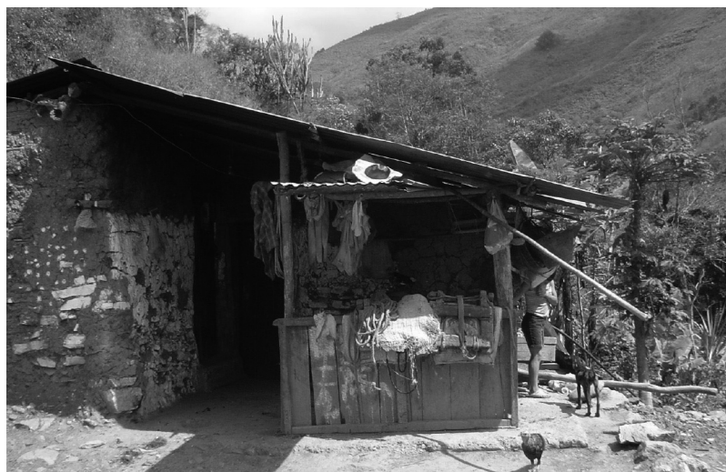
FIG. 1 Human dwellings conducive for transmission of Chagas' disease in endemic areas (rural area in Venezuela).
