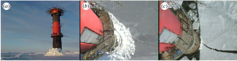
Figure 9. The Norströmsgrund lighthouse during ice action: (a) rubble formation after ice interaction (photo by courtesy of Basile Bonnamaire); (b) crushing ice failure and (c) splitting ice failure. (Online version in colour.)
