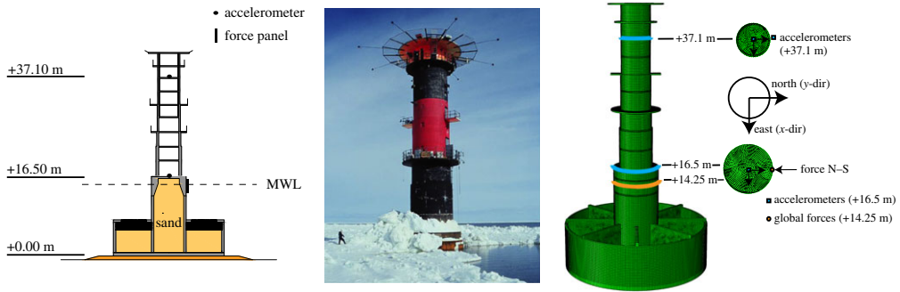
Figure 2. Illustration, picture and finite-element model of the Norströmsgrund lighthouse (from Nord et al. [26]). (Online version in colour.)
