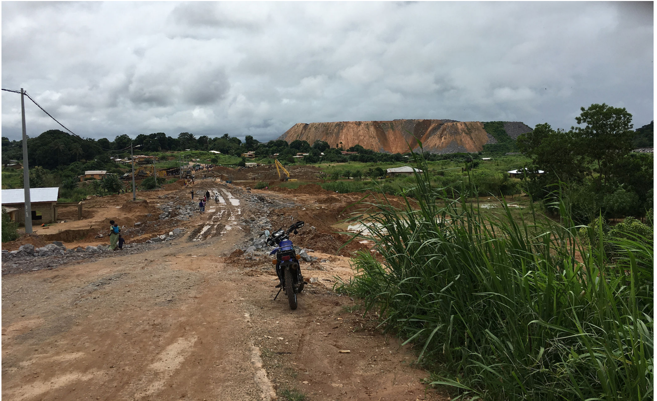
Figure 3. The Congo Town Bridge site after destruction, with Koidu Holdings' mine-tailings in the distance.
