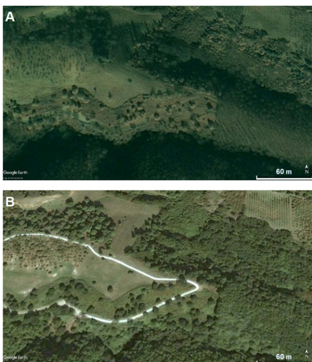
Figure 1. Comparison between two satellite images (between August 2004 (A) and November 2004 (B)) from Google Earth® constrains the timing of the construction of the reinforced concrete road.
