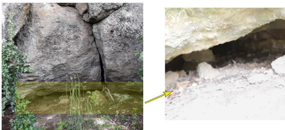
Figure 5. Images show how difficult it was to detect the entrance to the cavity. The magnified image on the right illustrates the inner part of the cavity beyond the obstructed access.
