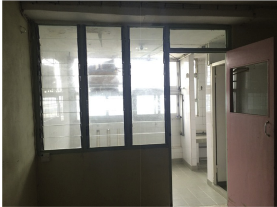
(a) The partition between the living room and the balcony
