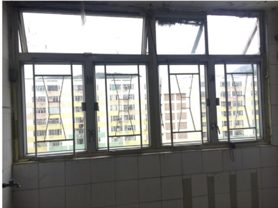
(c) The window and air slits on the external wall
