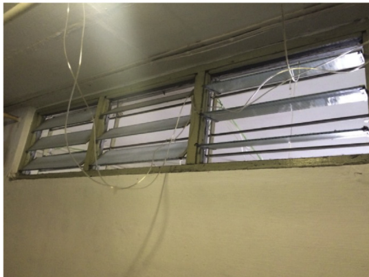
(b) The window on the internal wall near the corridor
