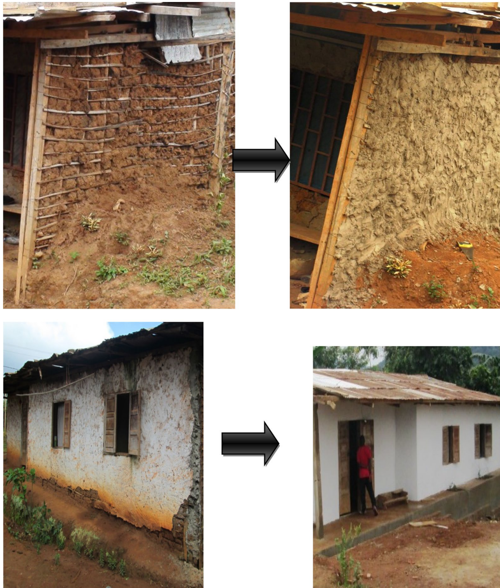
Fig. 6 Improvement on walls
