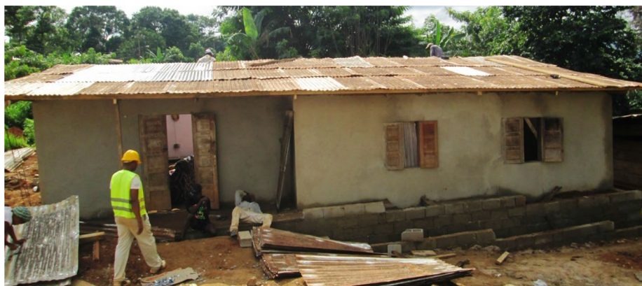
Fig. 7 Improvement on roofs
