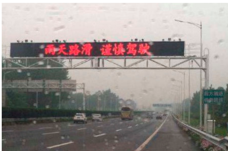
Figure 1. Variable message sign.
