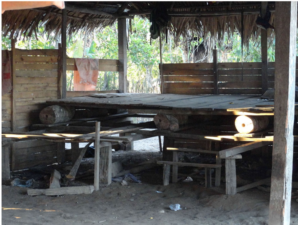
Fig. 6 A raft-type floating floor added to a house built in order to maintain a living space and protect belongings above the water line during the 2011 flood, which was both a high and long flood event. Note the height of the elevated floor, relative to the roof thatch; the logs below would allow the floor to adjust to changes in water elevation. (Photo taken by C. Abizaid in 2011)
