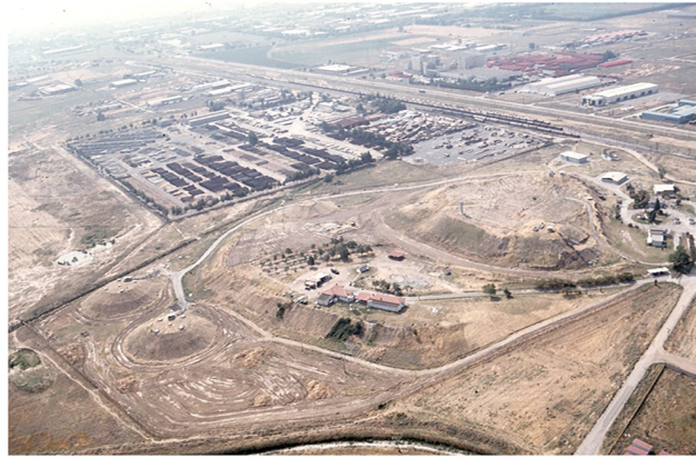
Fig 3. Aerial view of the tell-based settlement of Sindos, northern Greece comprising a higher and a lower artificial mound. The two conical structures to the left are modern (photo taken in 2001).
