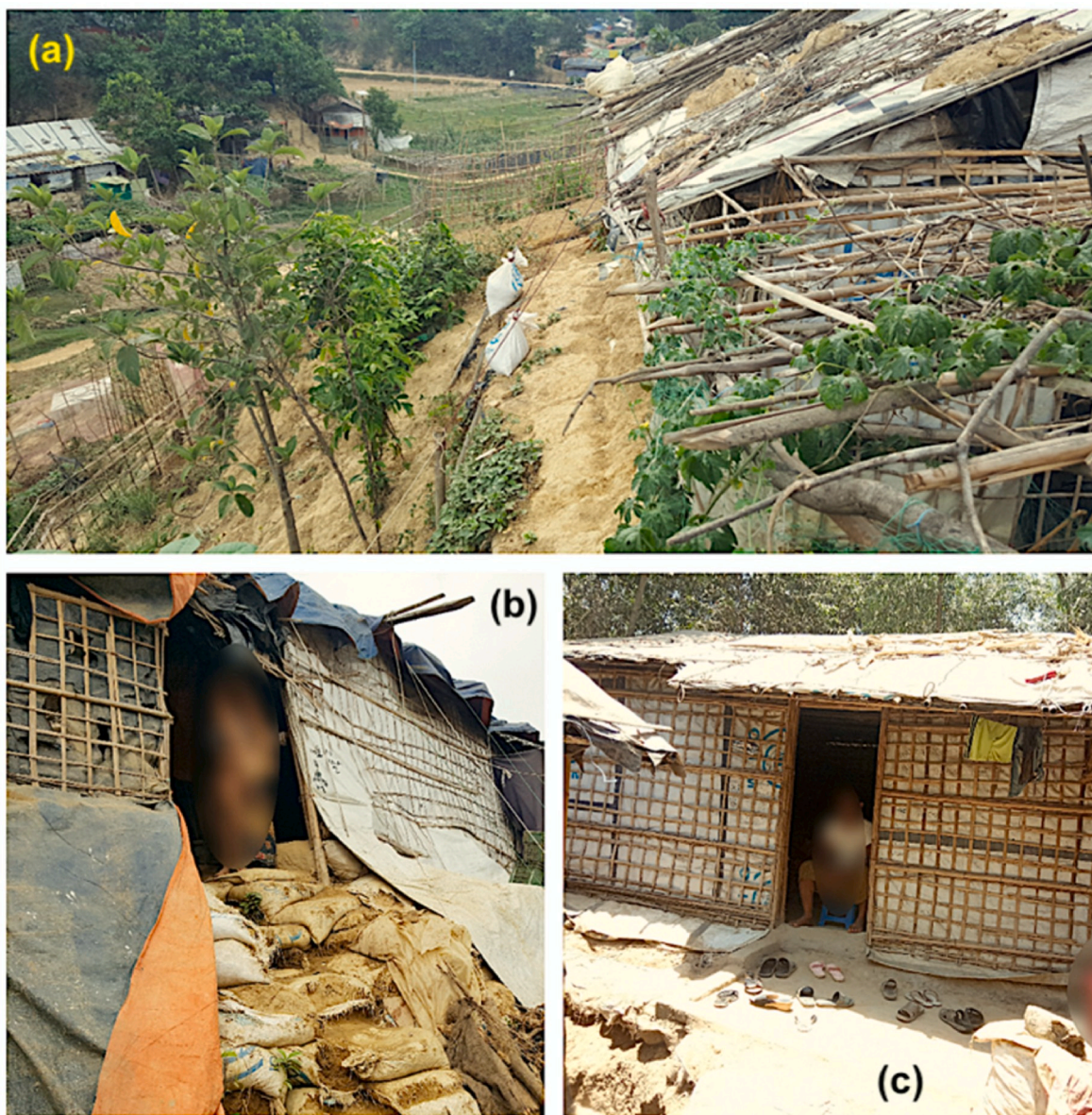
Fig. 7. (a) Use of tie-down ropes to protect the roof of shelters from uplifting forces, (b) placement of the sandbags at the edge of fragile shelters to minimise the risk of blowing during a windstorm, and (c) use of extra bamboos and plastic bags to reinforce the shelters from the monsoon rain (Source: Fieldwork, May 2019).
