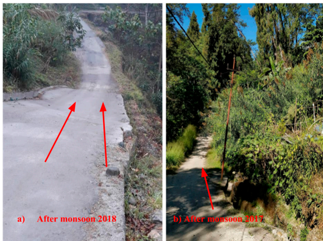
Figure 11. Displacements observed after 2018 and 2017 monsoons near sensor 2 (a) after the 2018 monsoon and (b) after the 2017 monsoon.
