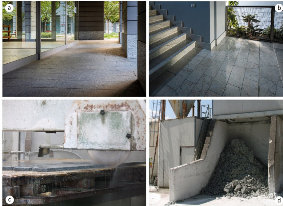
Figure 1. Typical installations of ornamental stones mainly containing alumino-silicate minerals (a) or carbonatic minerals (b); stone cutting process (c); stone waste powder resulting from the cutting process (d).
