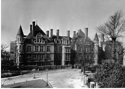
Fig. 4 National Institute for Medical Research—Hampstead (Front View). Source: Wellcome Library.
