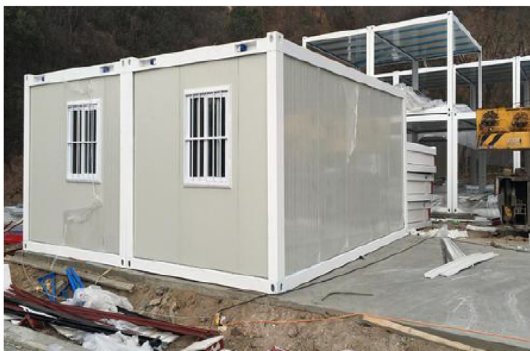
Fig. 9. Container-type prefabricated unit for the isolation ward. (Provided by China Construction Third Engineering Bureau Co., Ltd.)
