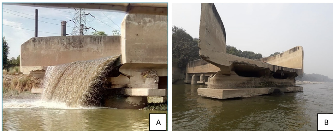
Fig. 15. Sisamau drain – the biggest source of untreated municipal wastewater (183.29 MLD discharge rate) in the Ganga River in the heavily polluted urban segment of Kanpur City, A: before lockdown (2019) B: during lockdown (2020).
