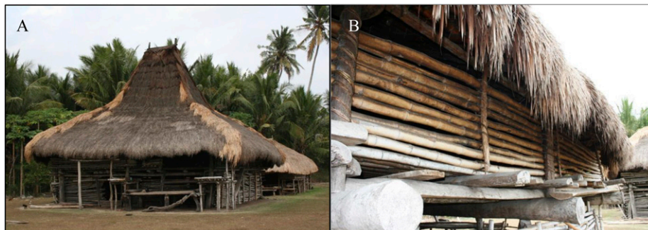
FIGURE 2. Traditional Sumba house structure (A) raised ~1 m aboveground and averaging ~70 m 3 in size with thatch roof, bamboo floors, and walls (B), which offer minimal protection from mosquito entry.
