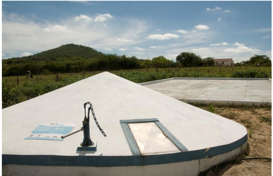
Fig 1. Boardwalk Cistern, a 52,000 liters water tank connected to a boardwalk that captures rainwater [16].
