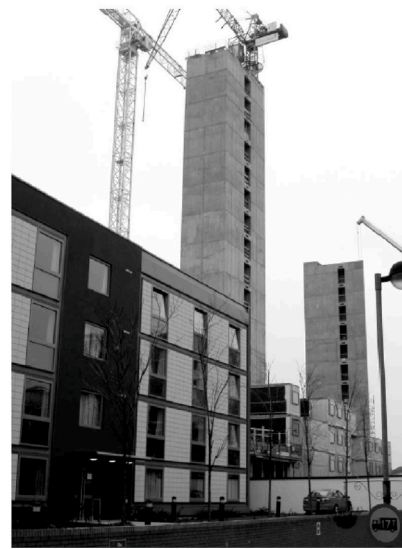
(c) 17-story residence in the UK [23]
