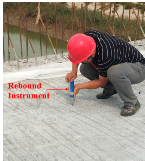
Figure 5. Test of the concrete strength by rebound instrument.
