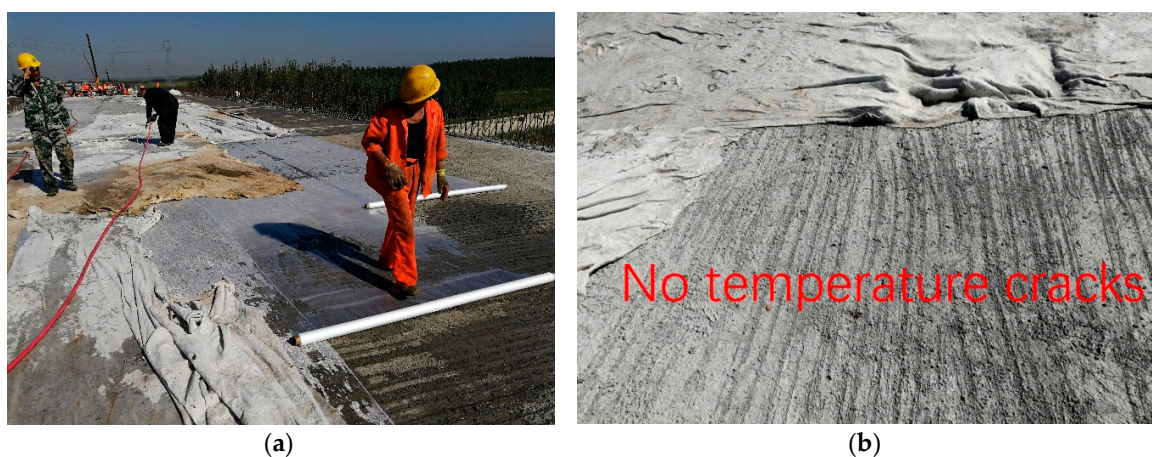
Figure 8. Photos of bridge deck: (a) curing; (b) 21 days after pouring.
