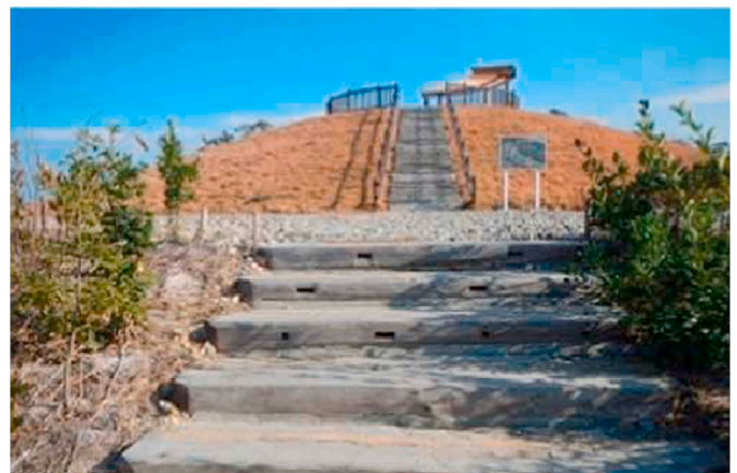
Fig. 9. Elevated ground in the disaster prevention park (also referred to as a vertical emergency shelter) [114].
