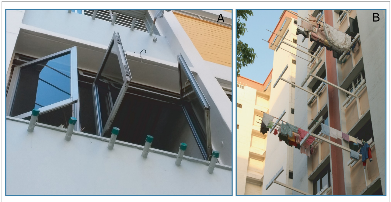
Fig 3. Redesign of washing line construction from bamboo pole holders with caps (A) to novel rack system (B).
