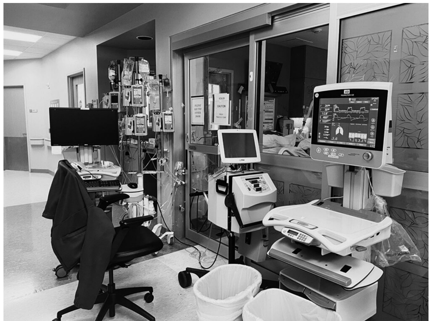
FIGURE 2 COVID-19 ECMO unit with mechanical ventilator, continuous renal replacement therapy machine, and IV manifolds, all located outside the patient room to minimize the need to enter the room. ECMO, extracorporeal membrane oxygenation
