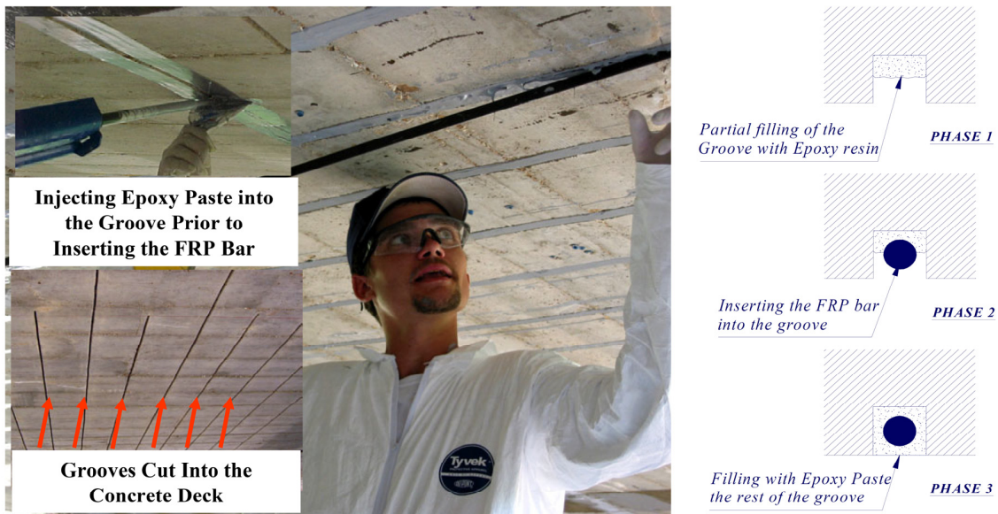
Figure 7. Implementation procedure for the prestressed NSM technique [72].
