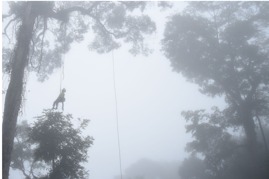
Figure 6. Installation of the canopy bridge by professional tree climbers, taken on 06 December 2015. Photograph taken by C.F.M.
