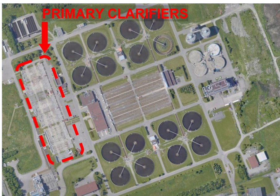
Fig. 1. Bird's-eye view of the Ottawa WRRF, with the primary clarifiers identified.
