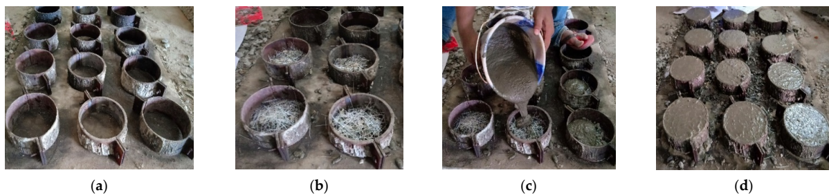
Figure 3. FPAFC casting process: (a) empty formwork, (b) packed fibres and coarse aggregates in formwork, (c) pouring of grout, (d) finished specimens.
