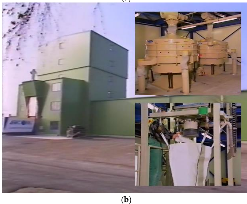
Figure 3. ERCOM installation for SMC/BMC (Bulk Molding Compound) recyclates: (a) scheme; (b) general view as well as sieving and packing hubs.
