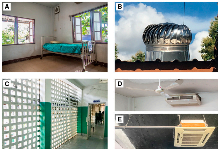
FIGURE 1. Environmental ventilation (photos by Dr. Rebecca Inglis). (A) Large, open windows on two different walls improve natural ventilation. The wall-mounted extractor fan should be set to blow outward not inward. (B) A whirlygig roof ventilator. The ventilator spins in the wind as warm air rises. The spinning draws out air from inside the building, improving ventilation. (C) Vented wall to increase airflow in a hospital corridor. (D) + (E) Two examples of split air system air-conditioning units in common usage and a ceiling fan. All three recirculate air within a room, rather than increasing the flow of fresh air from outside.
