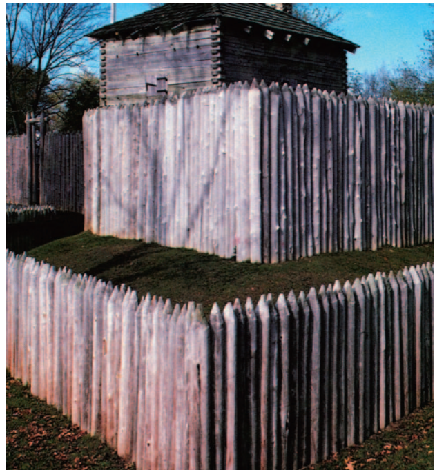
Fig 1. Photograph of the reconstructed 18th century Fort Massac in southern Illinois, demonstrating walls made of log palisades (courtesy of James P. Rowen).
