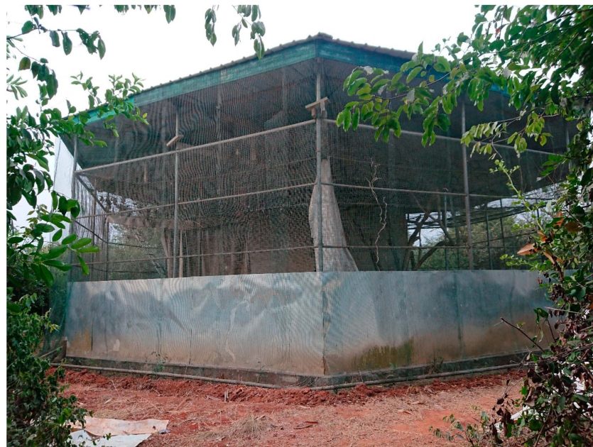
Figure 1. Cage housing the Eidolon helvum bat colony. The mesh double-walls, ground-level cladding and outer solid roof are clearly visible. Note, the bat colony can be seen roosting while hanging from the inner mesh roof towards the left side of this photograph.
