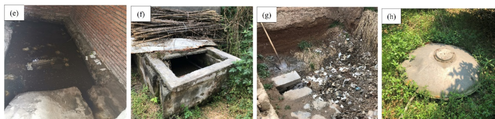
Collection and storage: e, f) Open-air storage for flushing toilet excreta, g) open-air storage for dry toilet excreta, and h) discarded biogas pool.
