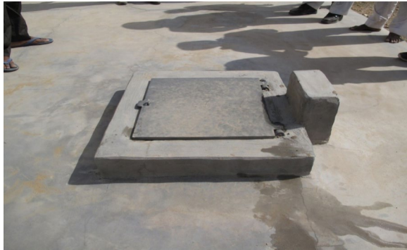
Fig. 2 Polyvinyl mosquito proof lid of size 45 × 45 cm
