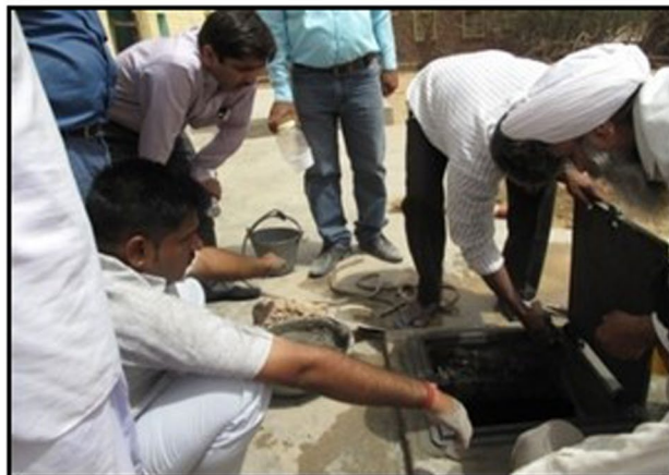
Fig. 3 Training/demonstration of process of replacement of tanka's lid
