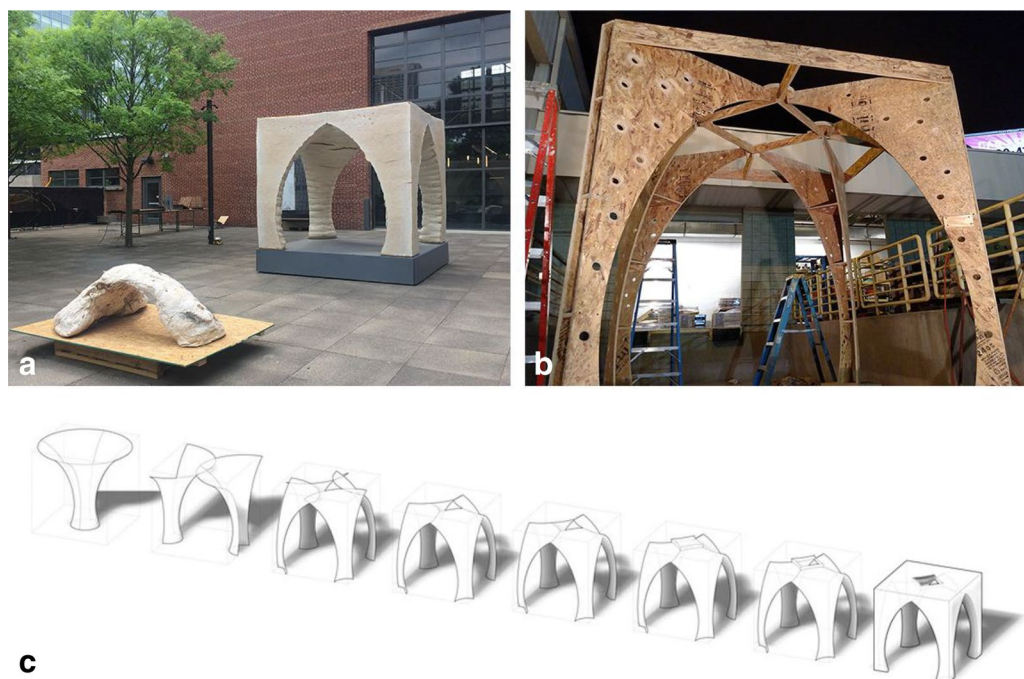
Fig. 6 a Perspective of the 'El Monolito Micelio' structure and another mycelium composite vault from the "Tactical Mycelium" series. Credit: © Jonathan Dessi-Olive. b The OSB supporting structural skeleton of the pavilion before the combination with the bio-composite. Credit: © Sean Miller. c Diagram showcasing the morphological development of the pavilion. Credit: © Sean Miller
