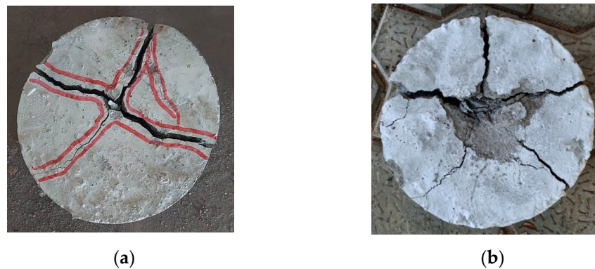
Figure 15. Typical failure patterns of the tested specimens under impact loading: (a) Non-fibrous specimen; (b) fibrous specimen.
